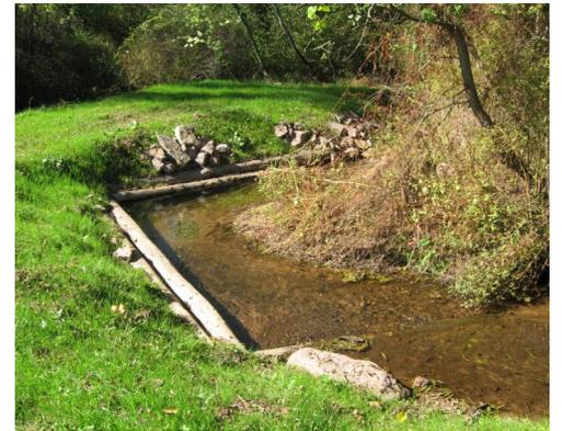
**A "mud sill" protects the stream bank and provides cover for fish.**
